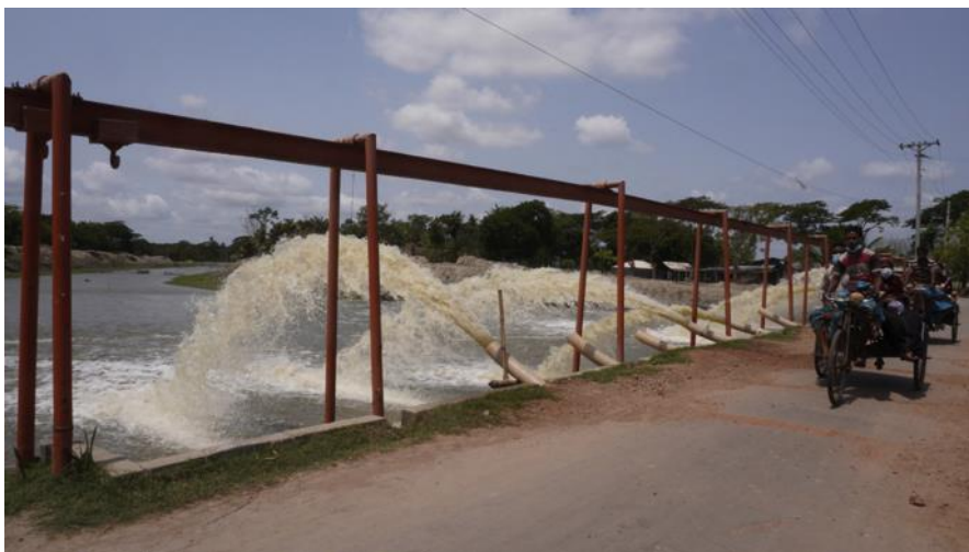
Picture-4.1.1.6: Pumping out water from the waterlogged area
