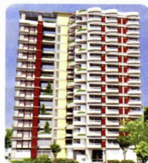
Tower 71 Manikdi, Dhaka Cantonment
