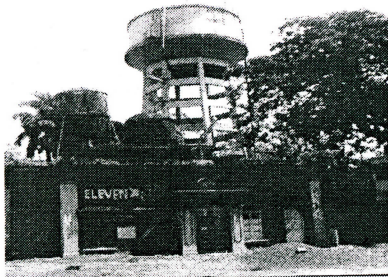
Photo 1: Iron and hardness removal plant
