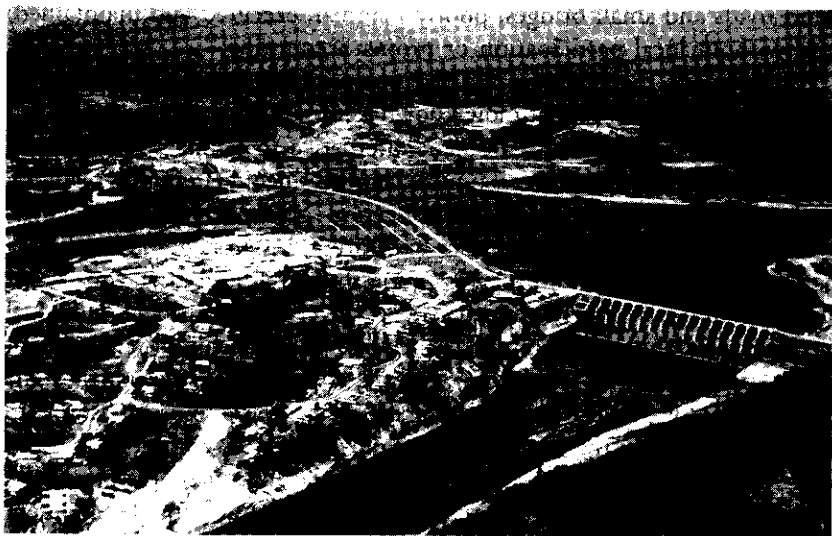
Plate 14.1. The Kaptai dam, 1964–5.
