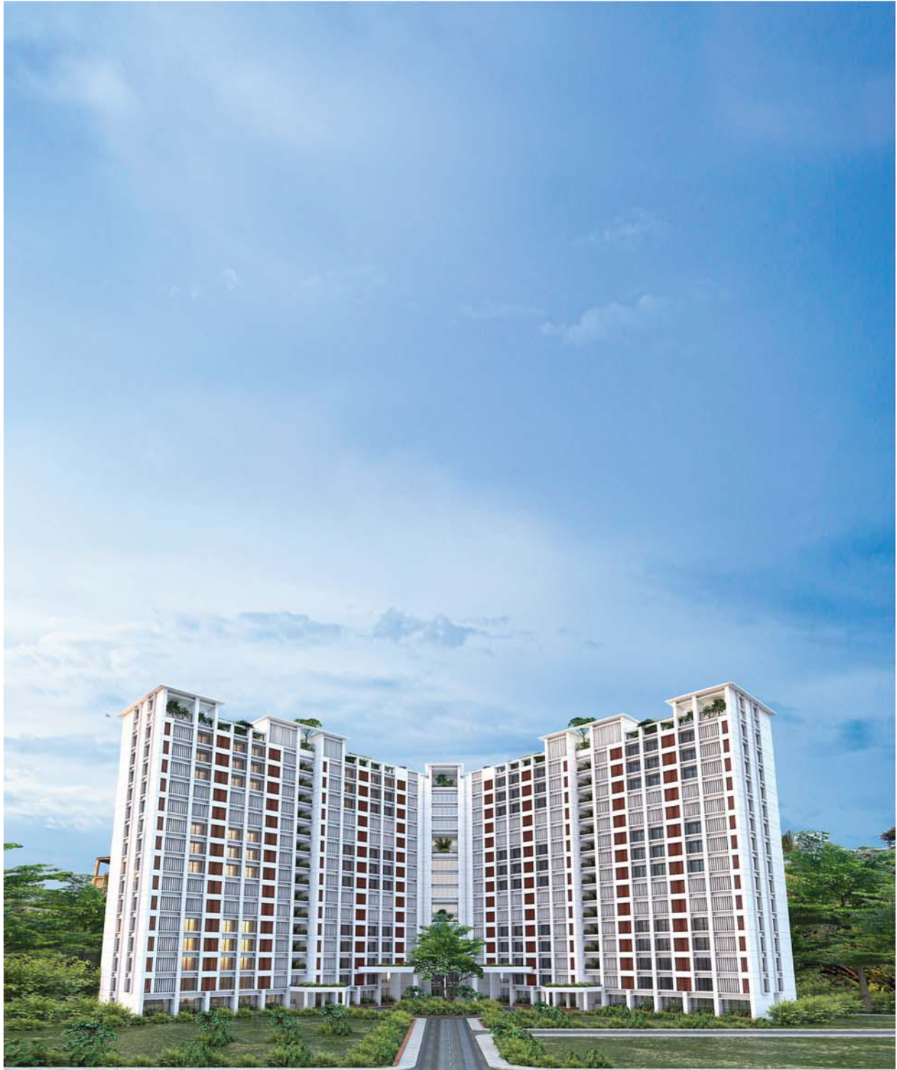
15 th Storied Dormitory Building, BPATC
