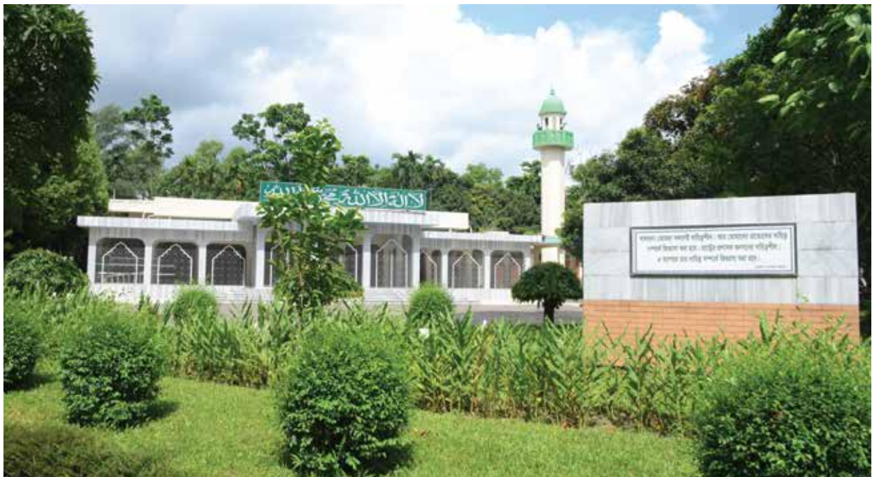
A view of renovated Mosque of BPATC
