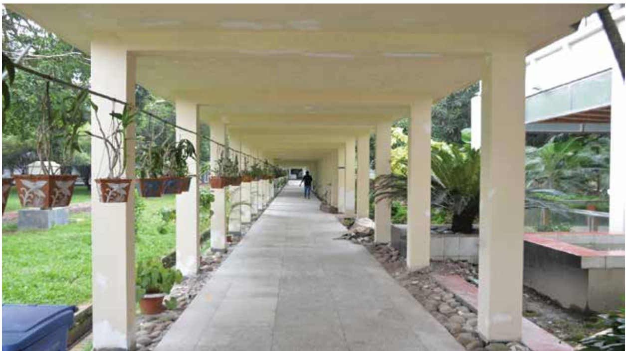
Renovated Corridor of the centre
