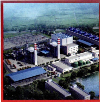
Shahjibazar 330 MW Power Plant Habiganj, Sylhet
