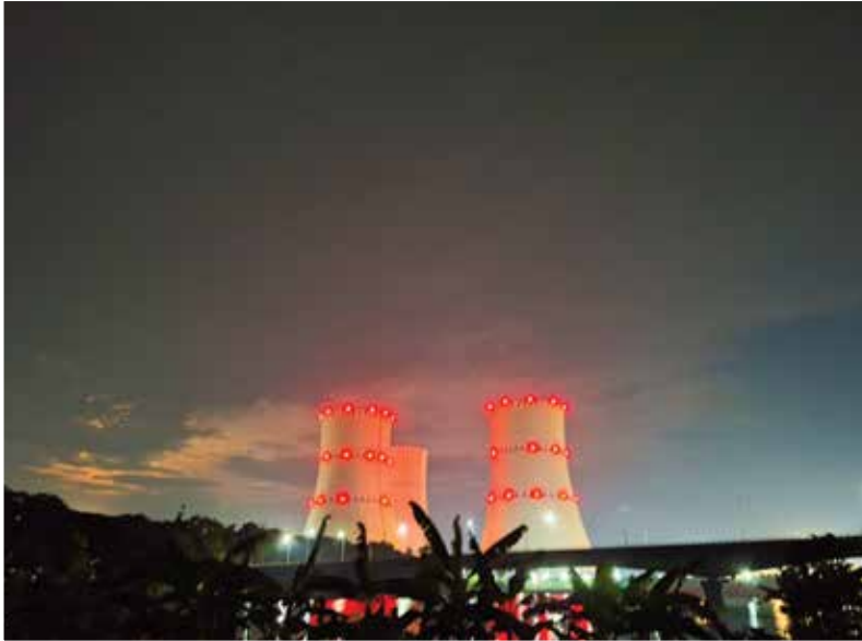
📷 Rooppur Nuclear Power Plant
