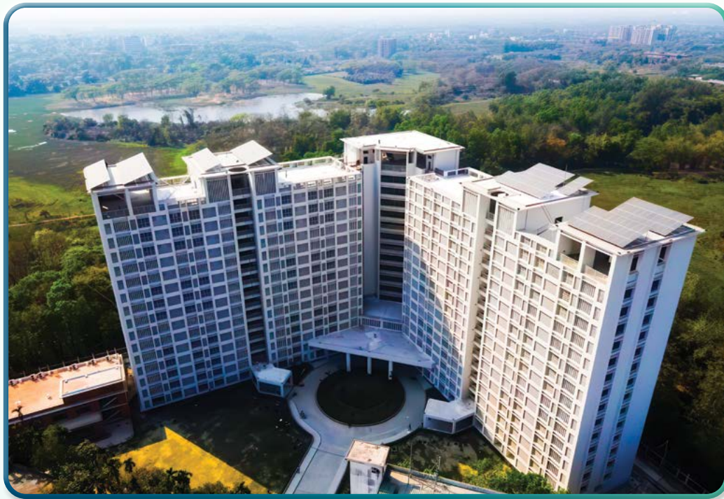
The iconic view of the 15 th Storey Dormitory, BPATC
