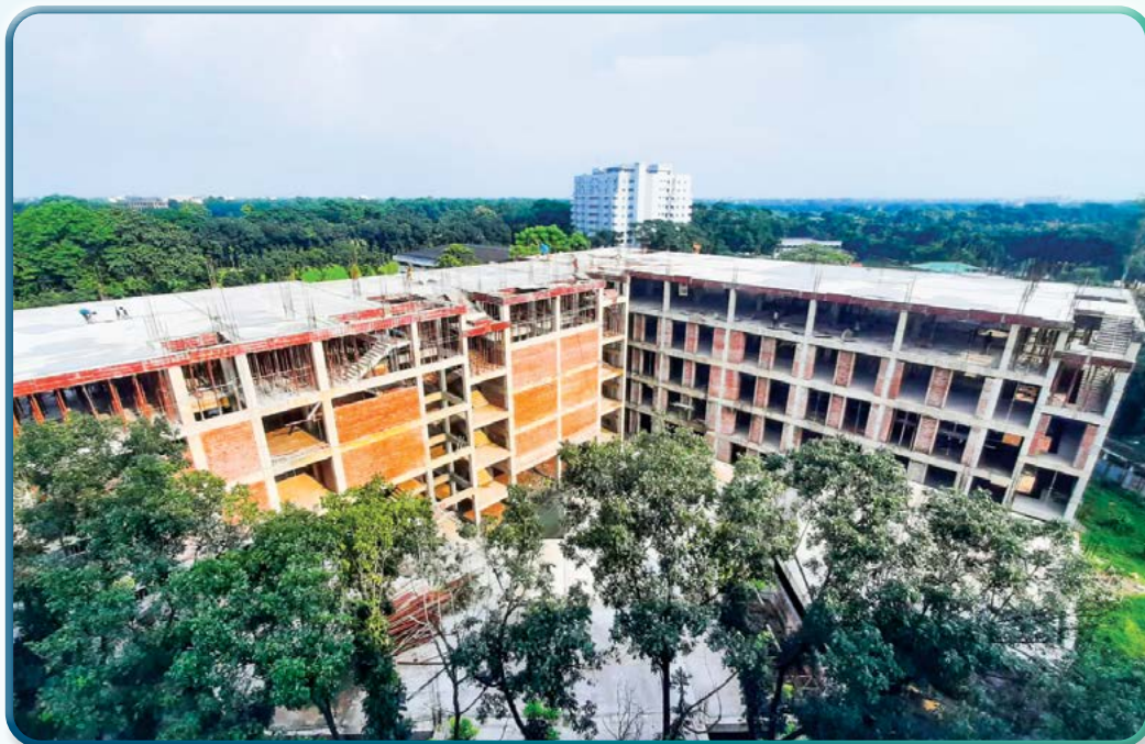
The modern five-storey cafeteria building nearing completion, designed to provide a spacious, well-equipped, and hygienic dining environment.
