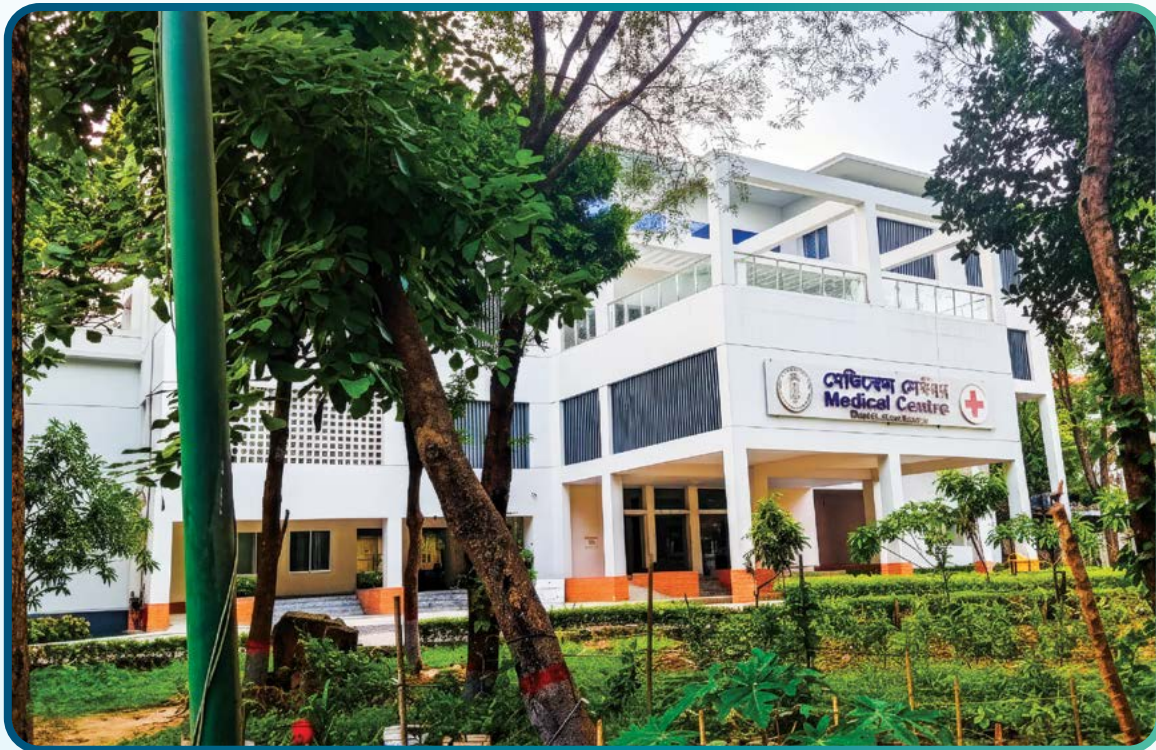
A closer view of the BPATC Medical Centre.
